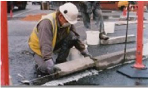
Polyester resin based material used for the bedding and fixing of kerbstones and precast barrier units to Macadam and concrete road surfaces. The product is supplied as a two pack system ready for onsite mixing, the mixed mortar will harden to give rapid strength gain reaching 25N/mm<sup>2</sup> in 2 hours. The bond strength, when adhering kerbstones or concrete units to roadways, will allow same day trafficking on trunk roads and estate roads
