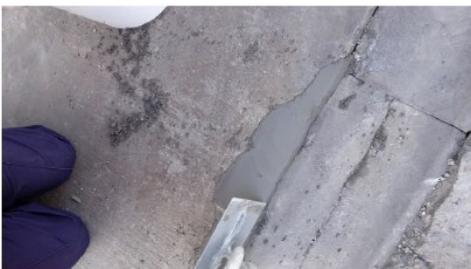
A two component product supplied as a pre-mixed Portland cement based non-shrink powder component plus a co-polymer latex gauging liquid. Highway Fastpatch can be used for repairs where rapid access and usage is required. The repair mortar enables a fair faced finish to be achieved and will give protection to exposed reinforcing steel. Working time is approximately 20 minutes and the mixed mortar, when placed, will harden in approximately 10 minutes.
